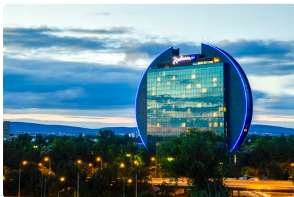
Radisson Blu Hotel, Frankfurt with large-scale hydrogen fuel cell installed
