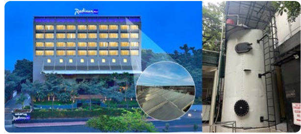
Radisson Blu Hotel, Bengaluru Outer Ring Road which is the first LEED ZERO CARBON certified hotel in Radisson Hotel Group's global portfolio including a photo of the biogas installation
